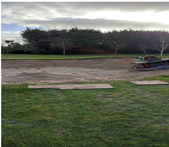
Spreading and compacting the face.
