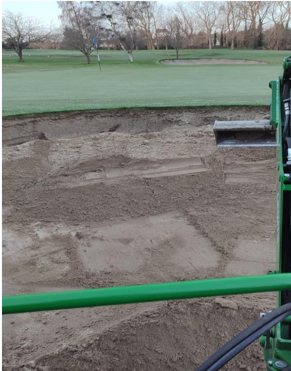
Stripping out the old sand.
