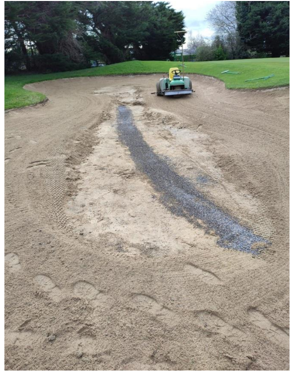
Drainage repaired and old sand replaced
